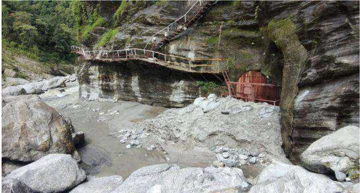
Figure 5: Water supply intake gate was disrupted by the Melamchi Flood
