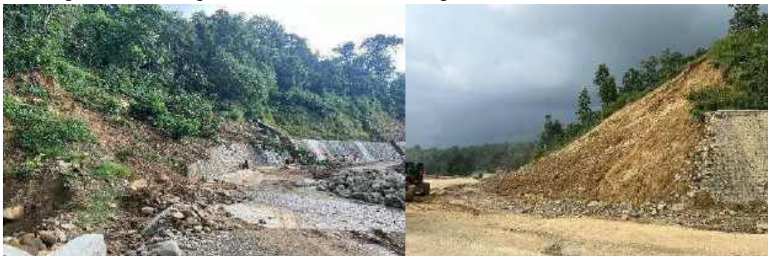
Figure 1: Photographs showing active landslide along Daunne road section.
