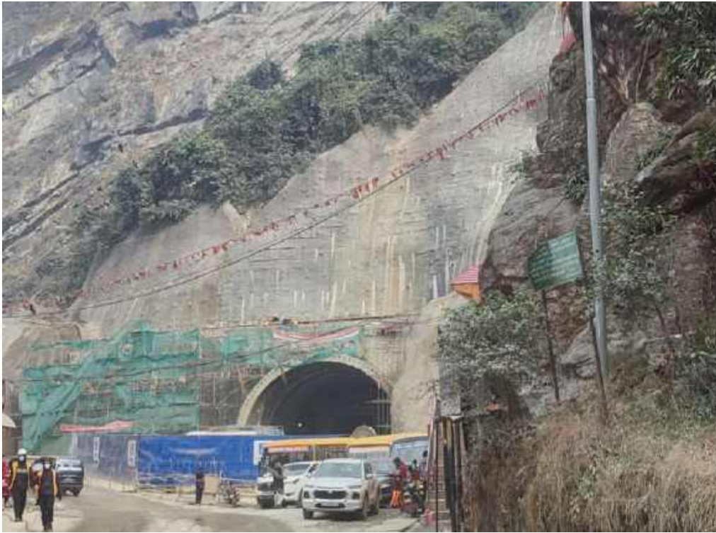
Figure 5: Photograph showing south portal of Siddhababa road tunnel
