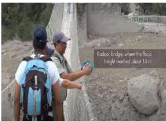
(a) 15 m height of suspension bridge destruction
