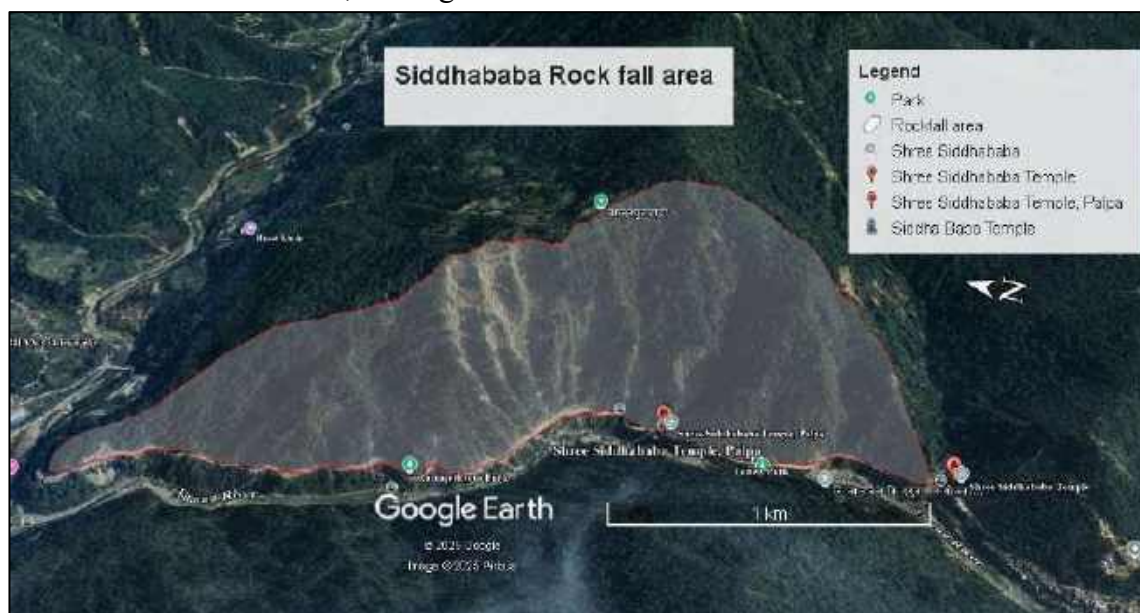
Figure 1: Photograph showing Siddhababa rockfall area in the shaded zone
