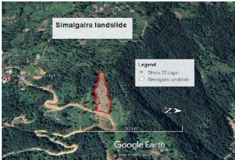
Figure 1: Photograph Showing Simalgaira landslide in 2076
