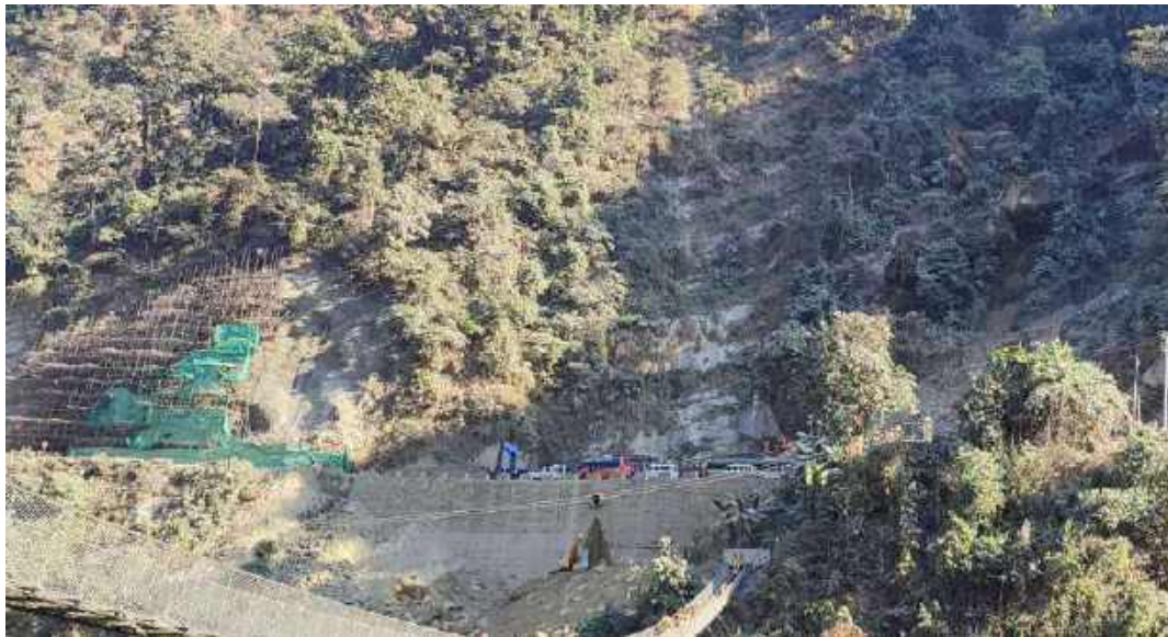
Figure 6: Photograph showing northern portal of Siddhababa road tunnel
