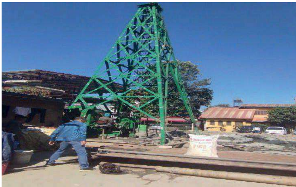
Figure 1: Direct rotary drilling method in Jawalakhel
