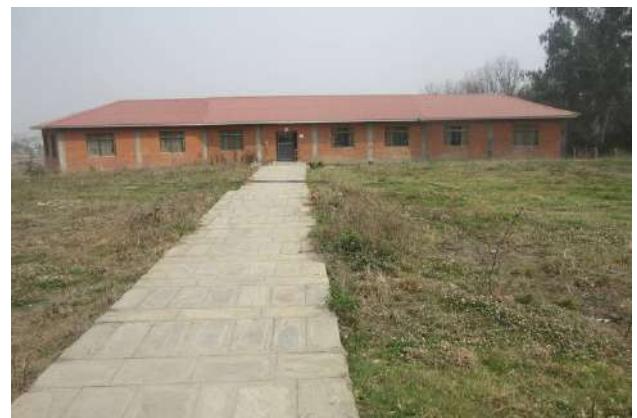
New building for laboratory
