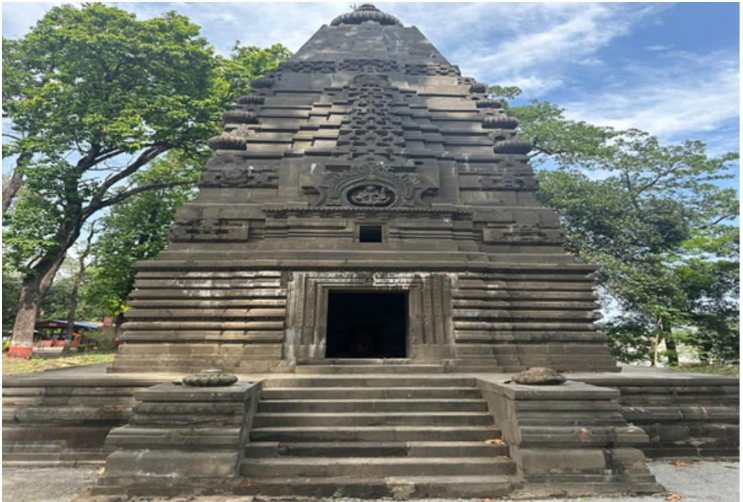
Fig. 5: Mahadevathan located at Sikhrauli
